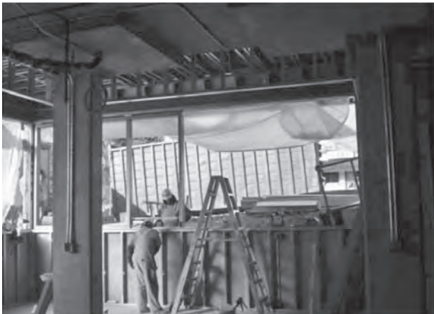
Installing windows in the Bookstore
