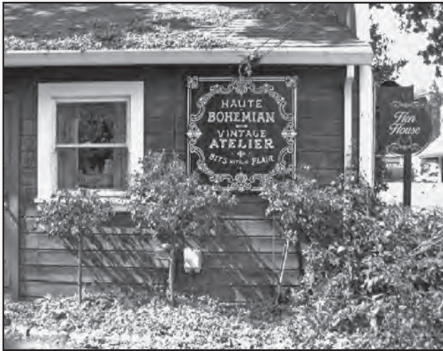
Hen House, building detail as it looks from the south side of the building.
