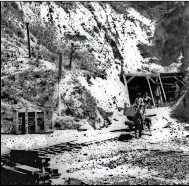
Excavating the Tunnel
